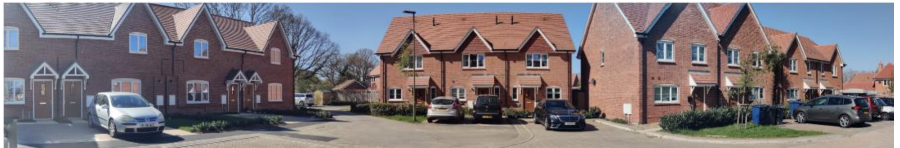
Photo 7: Horsham Road Phase 1, Cranleigh
