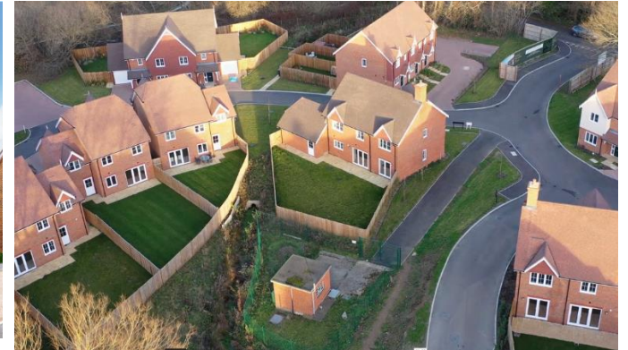
Photo 6: Weyburn Works, Elstead
